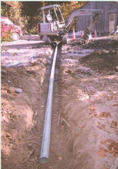
The Laurie Storm Sewer Replacement project completed last year and this spring increased the Township's total flood alleviation grant and township matching dollars spent since 1992 to approximately \$4,698,000. This \$323,000 project involved the installation of larger storm pipes in order to alleviate upstream flooding and sinkholes along Laurie Drive. An Issue I grant for \$271,000 funded 84% of this project.
